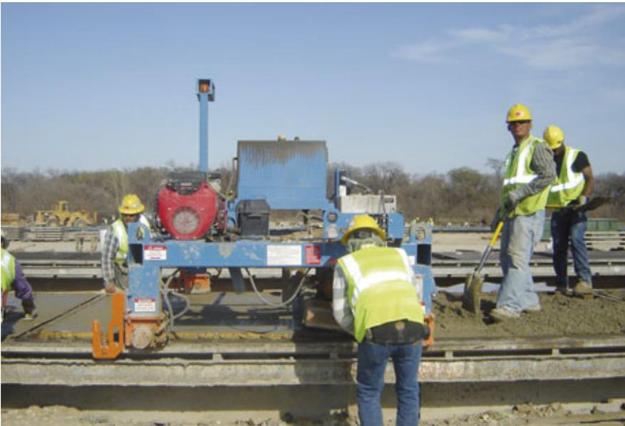
Controls for the finishing machine are located along the side for easy access.
