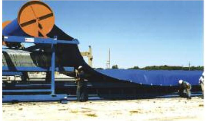
**Carts help protect your investment in insulated blankets and tarps by keeping them off the ground and neatly rolled when not in use. Two men can quickly and easily cover and uncover a bed, saving time and labor.**
