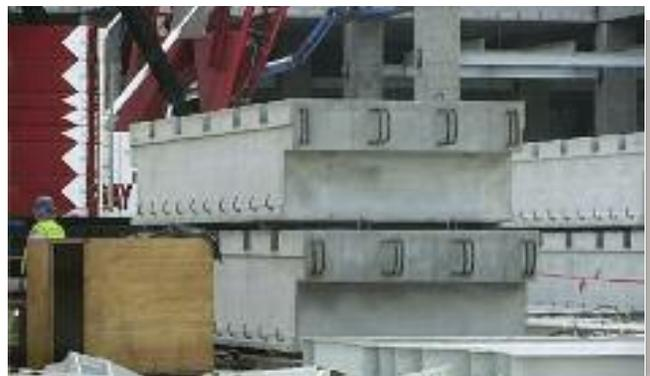
The waffle slabs delivered by Unistress Corporation are enormous, weighing as much as 24 tons each.
