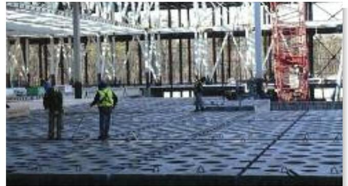
The waffle slabs form the floor of the clean room for the new semi-conductor manufacturing facility.
