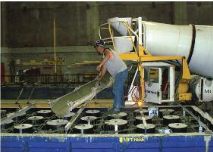
The use of SCC made pouring more efficient and contributed to a better finish.
