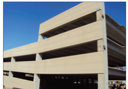
Coreslab is casting 60 foot spandrels on its new self-stressing casting table.
