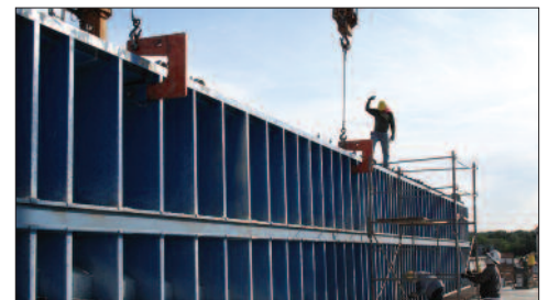
Vertical lifting apparatus for handling sideforms
