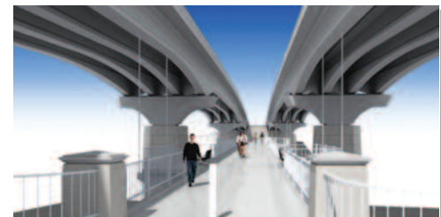
Suspended pedestrian bridge
