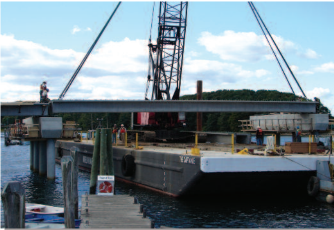
Bridge over the York River on Route 103 in York, Maine.
