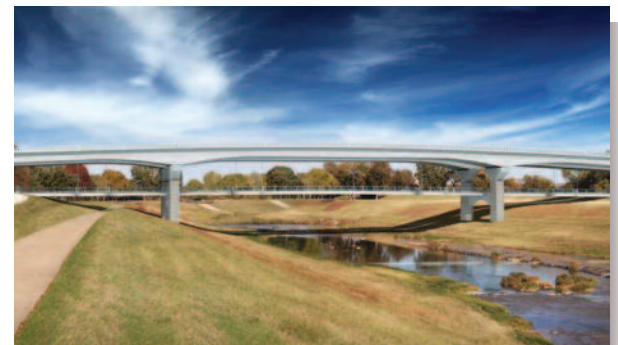
Clearfork, Main Street Bridge
