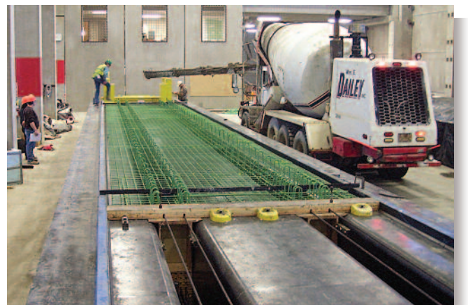
W.E. Dailey, Non-Self-Stressing NEXT Beam Form
